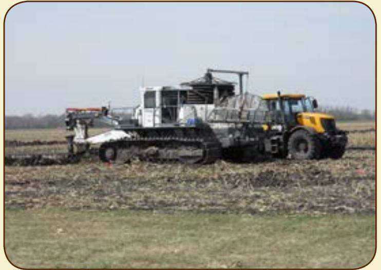
The tile plow installed drain tile this spring.
