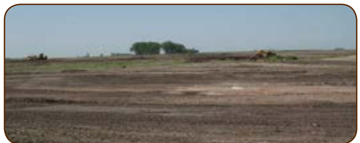
Leraas gravel pit reclamation.
